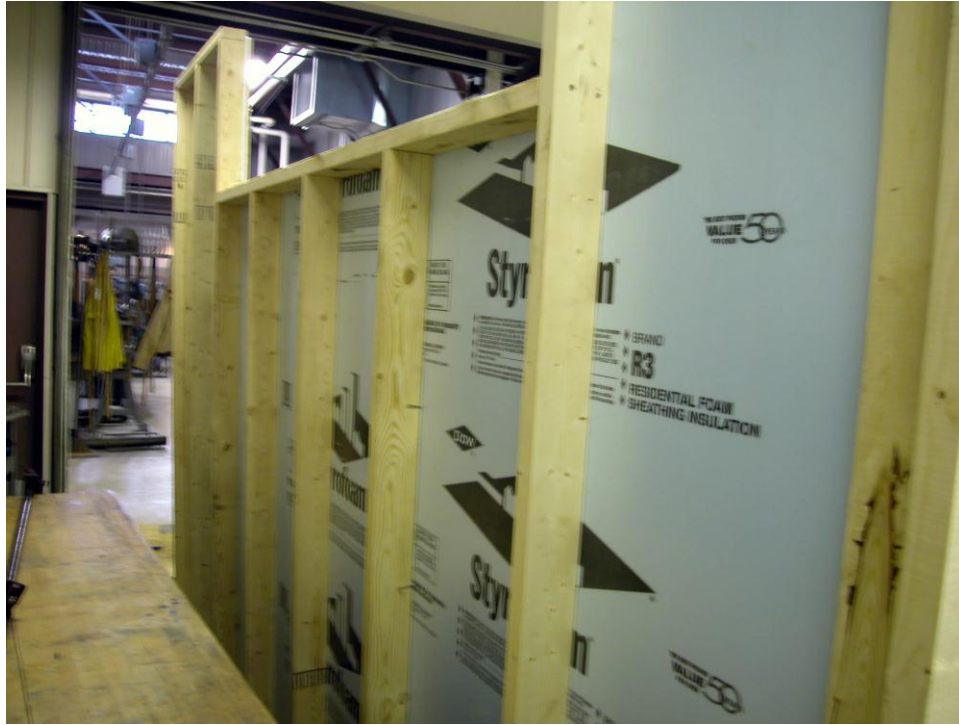
Figure 31. Photo of one of the dehydrator walls during construction.
