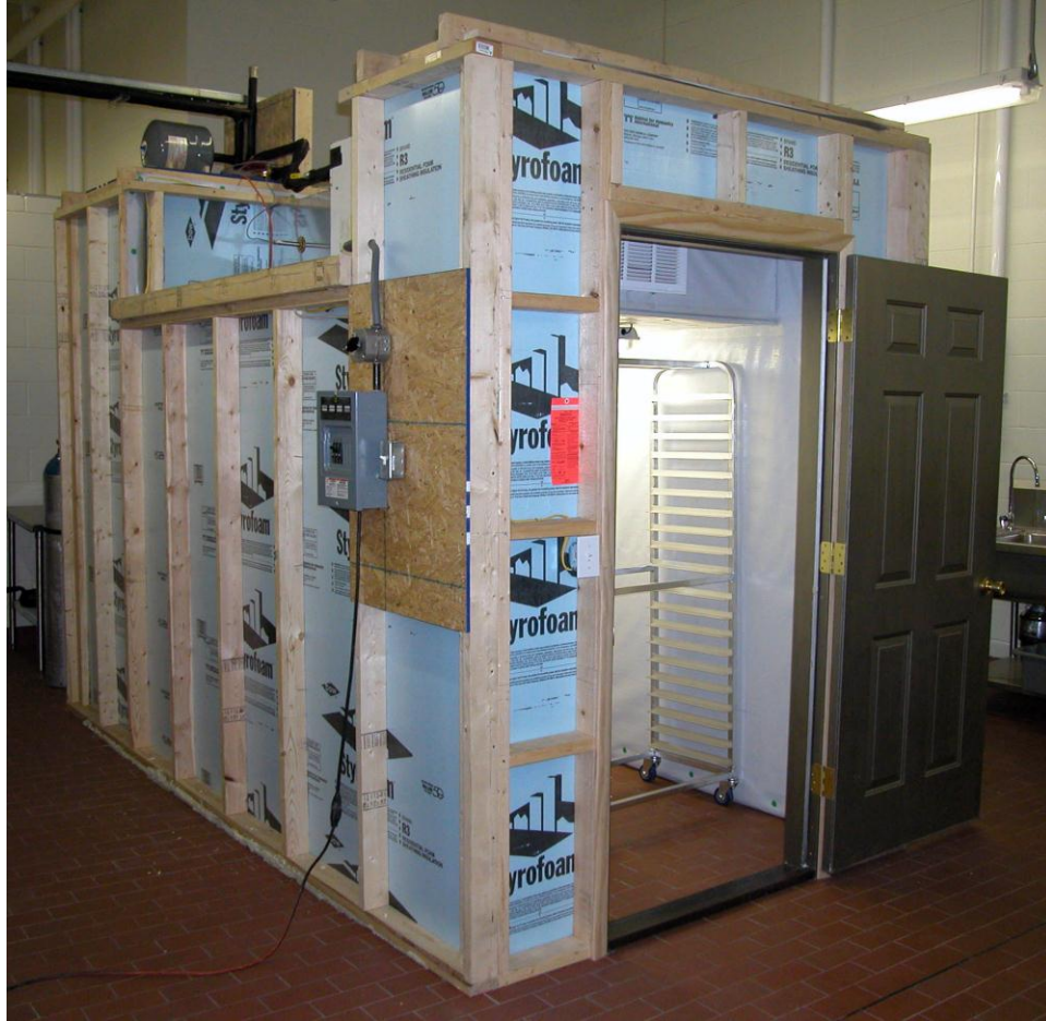
Figure 30. Photo of the nearly completed dehydrator
